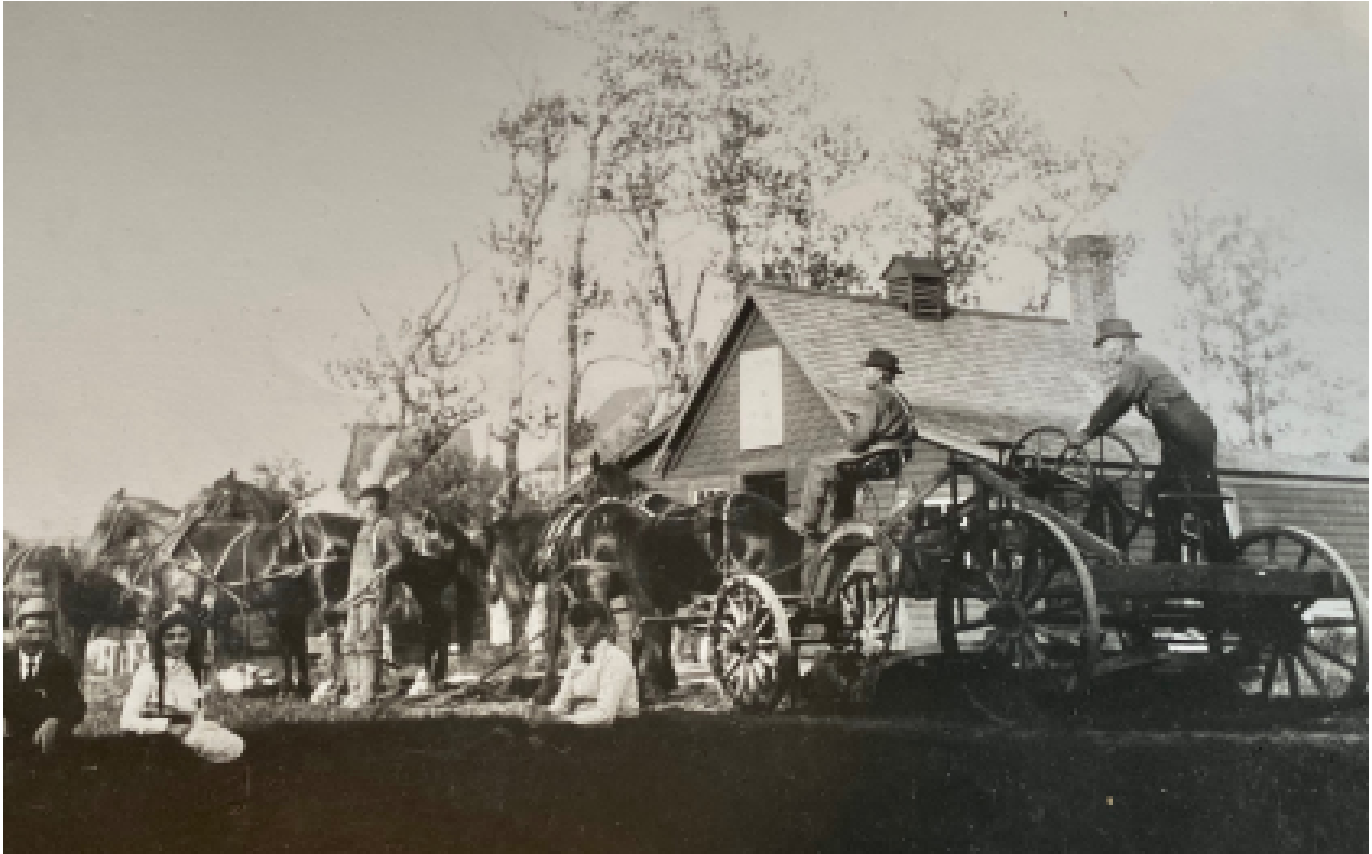
Clarence Turner and road crew circa 1910. Blacksmith shop is in the background.
